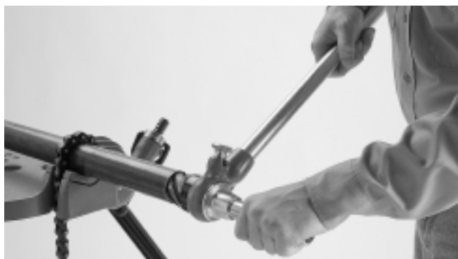
Figure 2 – Reaming End of Pipe
