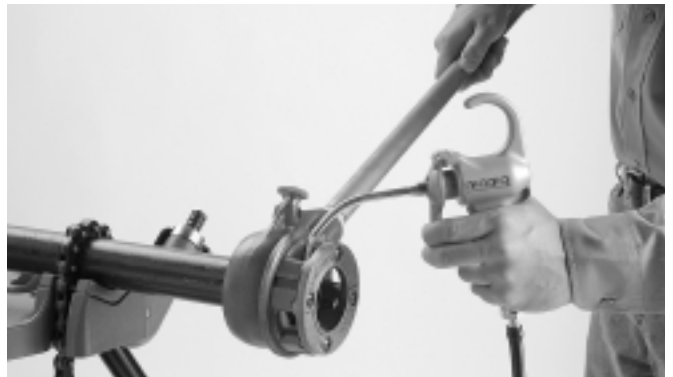
Figure 4 – Applying Thread Cutter Oil
